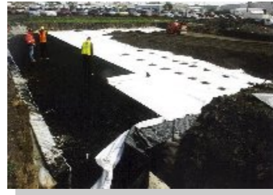
Completed 620 cm tank Note: compaction with 3 tonne roller
