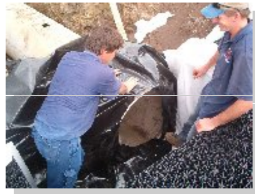
Penetration of 750mm pipe through Damtuff liner
